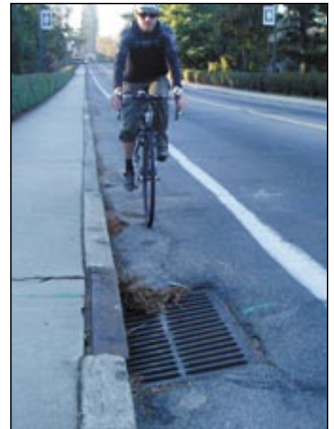
Figure E.3 - One of many dangerous drainage grates that exist around Durham
