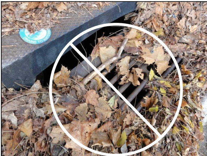
Storm drains lead directly to streams. Too many leaves in streams are bad for water quality. Plus, leaves clog the drainage system and can cause flooding. Always remove leaves from the street, storm drains, and ditches.
